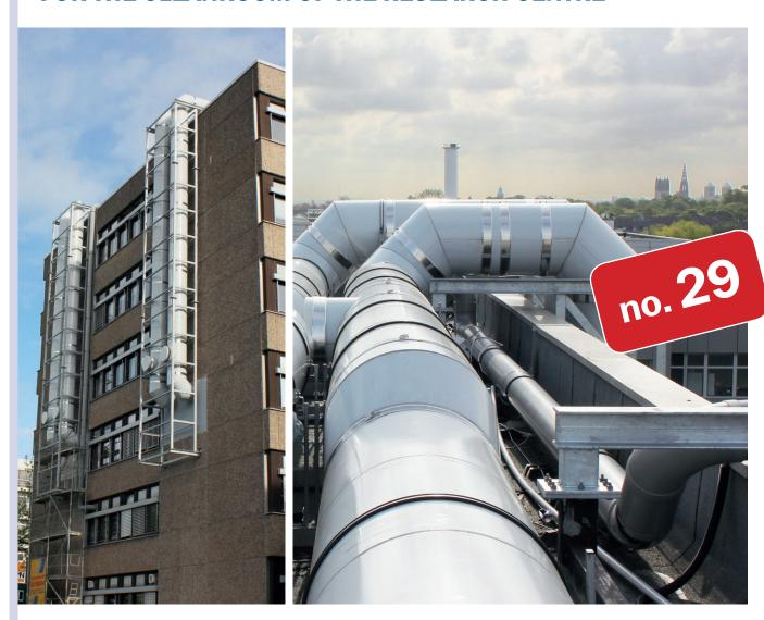
Design and implementation of an air duct system with statically appropriate attachment to the facade
