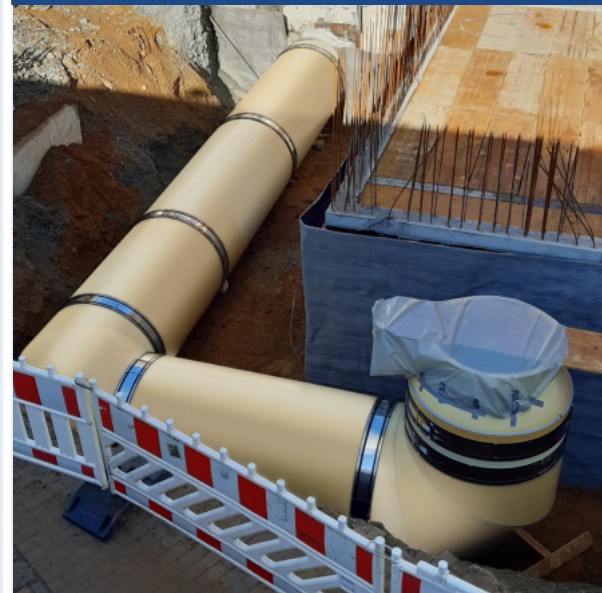
Planning and realization: within the building the LAVANTUS® air duct is connected to a rectangular duct, the ventilation tower is installed later.
