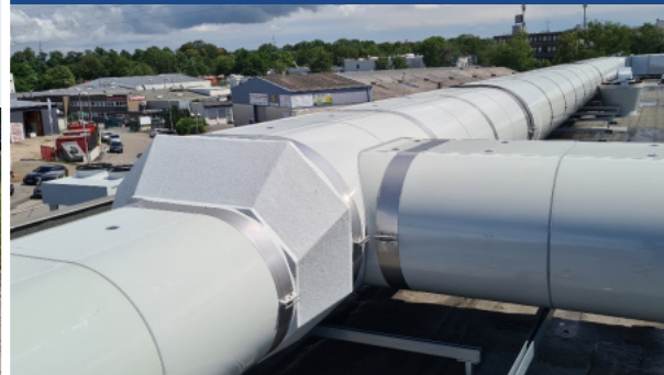
Our technicians proudly present their "giant babies": custom-made special components, in this case reductions of various diameters
