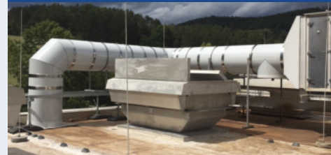
After: clean solution with air ducts made of PUR rigid foam and GRP
