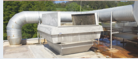
After: clean solution with air ducts made of PUR rigid foam and GRP
