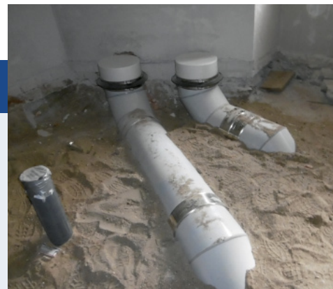
Underground installation inside and wall duct to the outside
