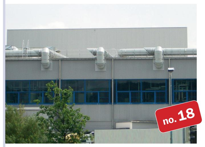
Air duct system with pipe dimensions of 920 mm, installation inside and outside the production hall
